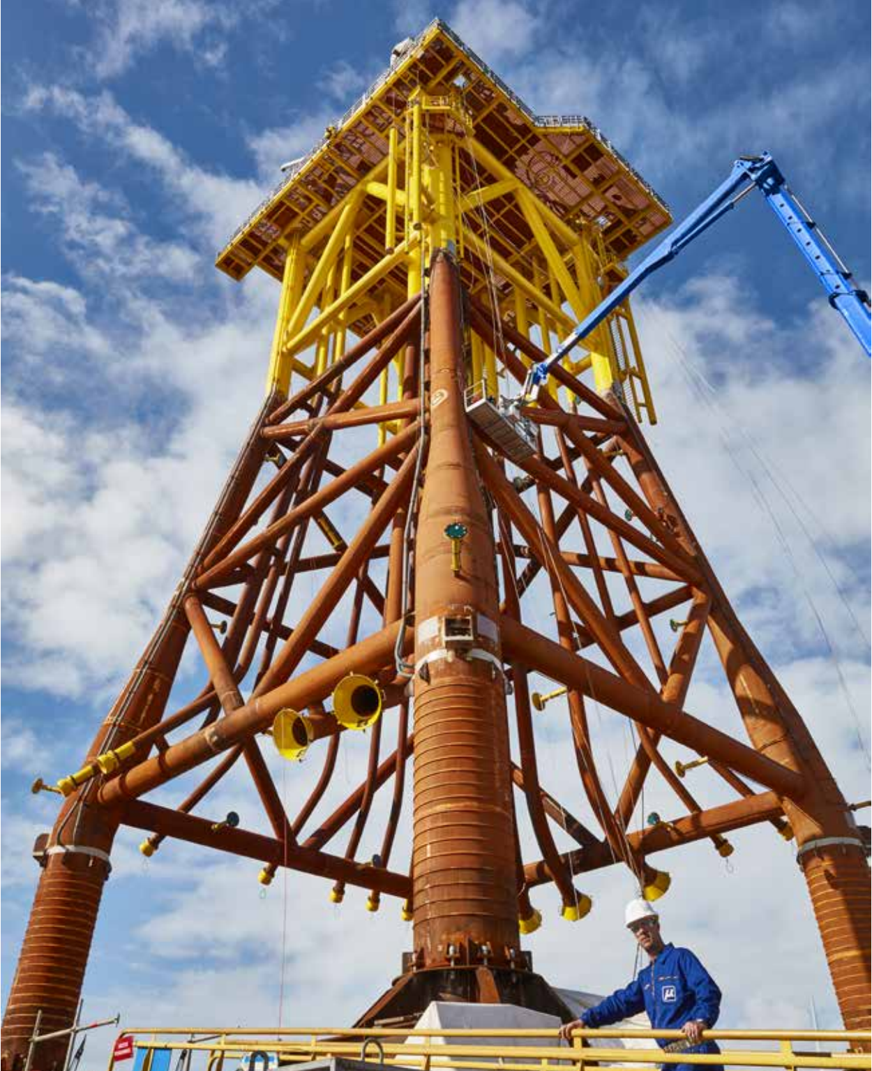
Jacket construction for offshore wind power station in Saint-Nazaire, France
